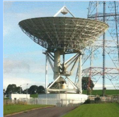
Ireland Elfordstown – handed over 2011/05
